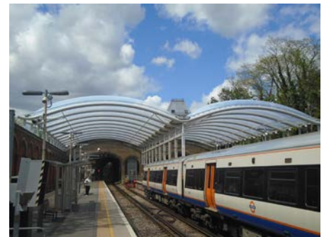
The completed roof
