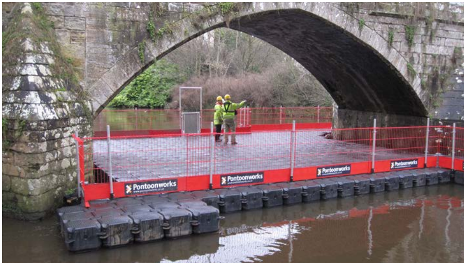
The 700m 2 pontoon was able to float two six-tonne excavators
