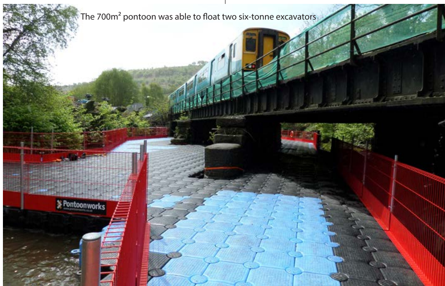
Pontoonwork’s engineering access solution on the River Cynon in Wales
