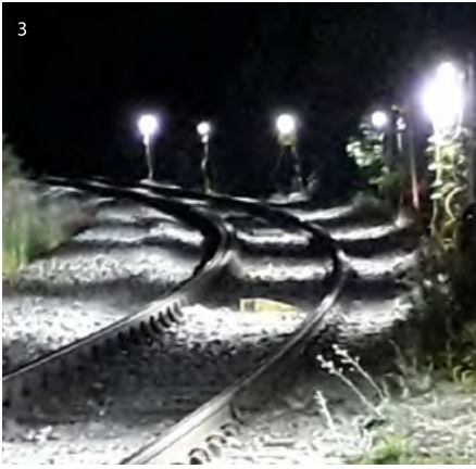
Examples showing light 'striping' with light and dark patches using traditional diesel powered lighting
