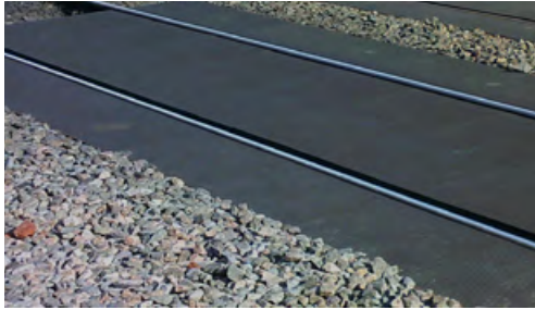
Semi-Permanent RRAP's /Temporary Level Crossing
