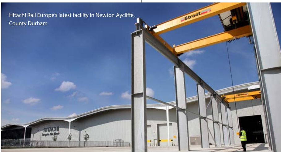
Street Crane also has lifting equipment at Edinburgh Tram's depot
